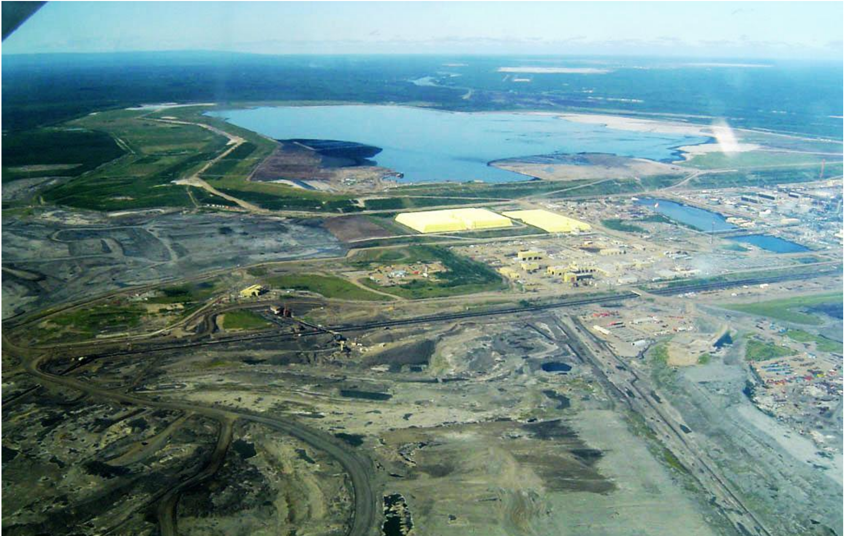
Syncrude Tailings Dam - Mildred Lake
